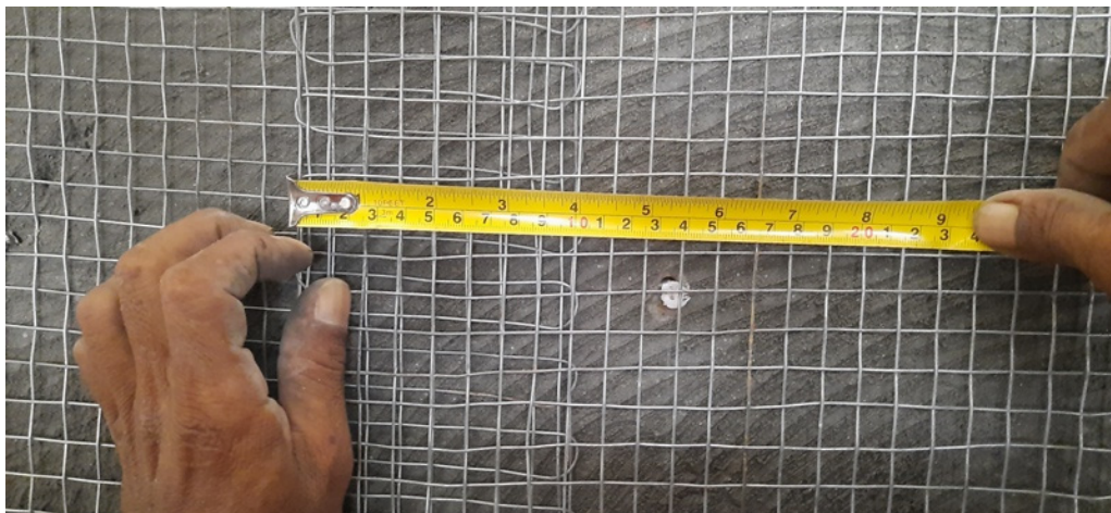
Figure A.2.18: Checking the lap length of wire mesh-100 mm
