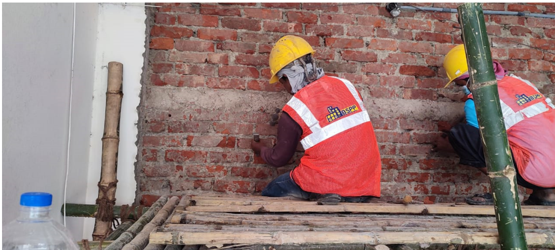
Figure A.2.5: Plaster removal for brick joint
