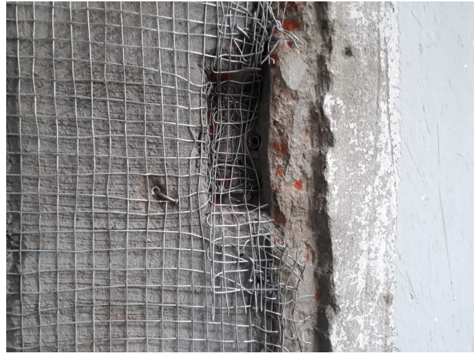
Figure A.2.50: 75 mm wire mesh lapping before installation of angle (only where the thickness is inadequate)
