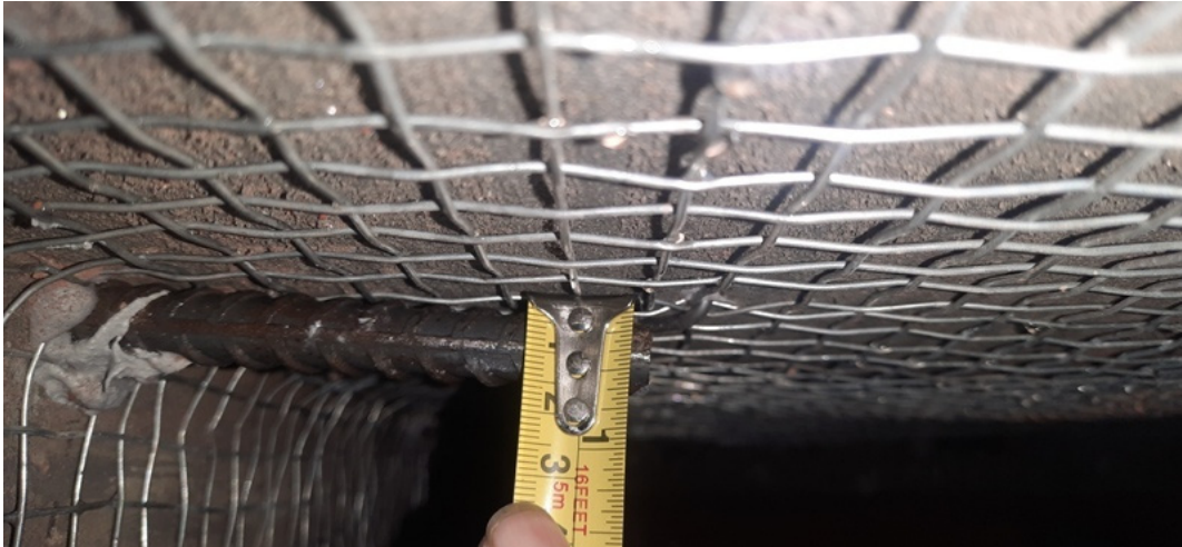
Figure A.2.24: Checking the minimum length required for final mortar work to cover dowel.
