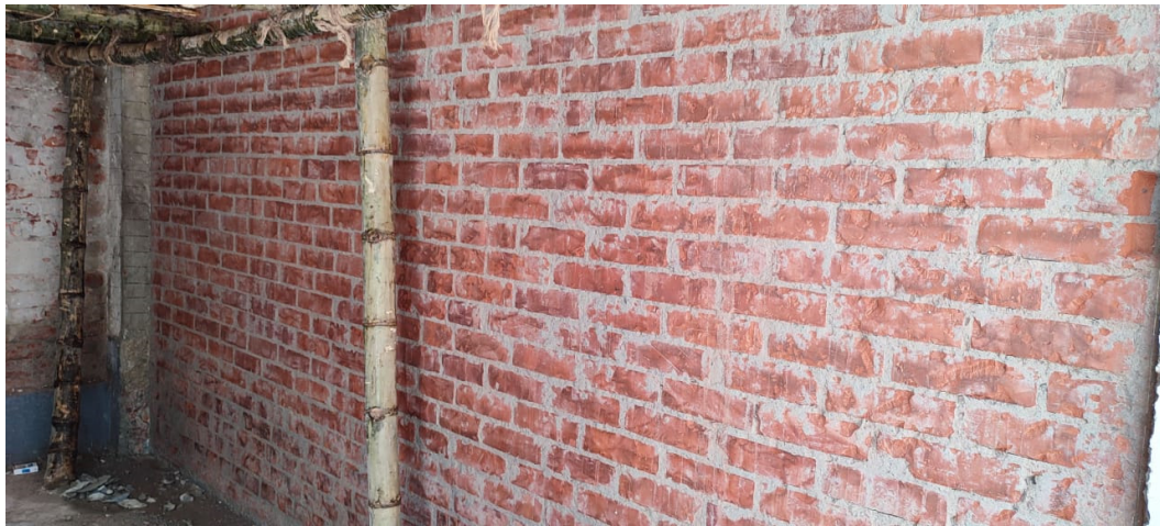
Figure A.2.38: Prepared surface for ferrocement mortar work
