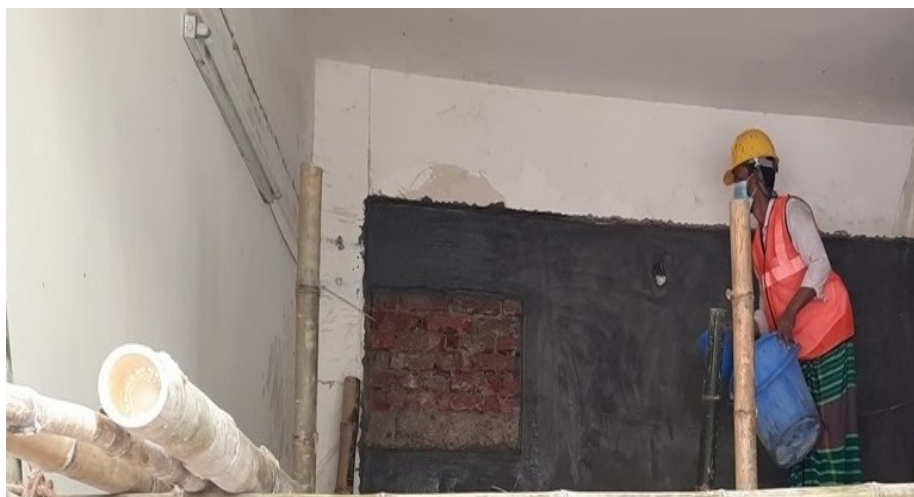
Figure A.2.12: Spreading water for curing work
