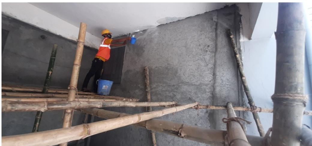
Figure A.2.66: Continuous 7 days water spreading for curing work
