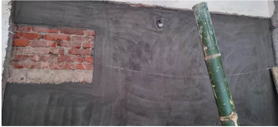
Figure A.2.10: 10 mm mortar work without wire mesh (locally known as rough plaster)
