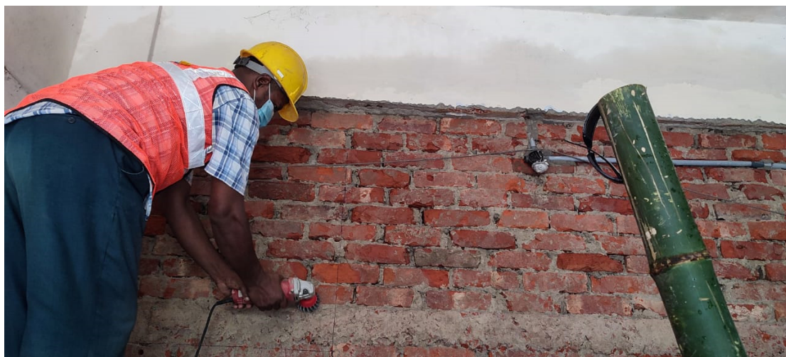
Figure A.2.6: Cleaning brick surface with steel brush
