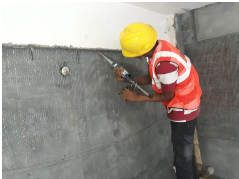
Figure A.2.21: Injecting epoxy resin to install dowel
