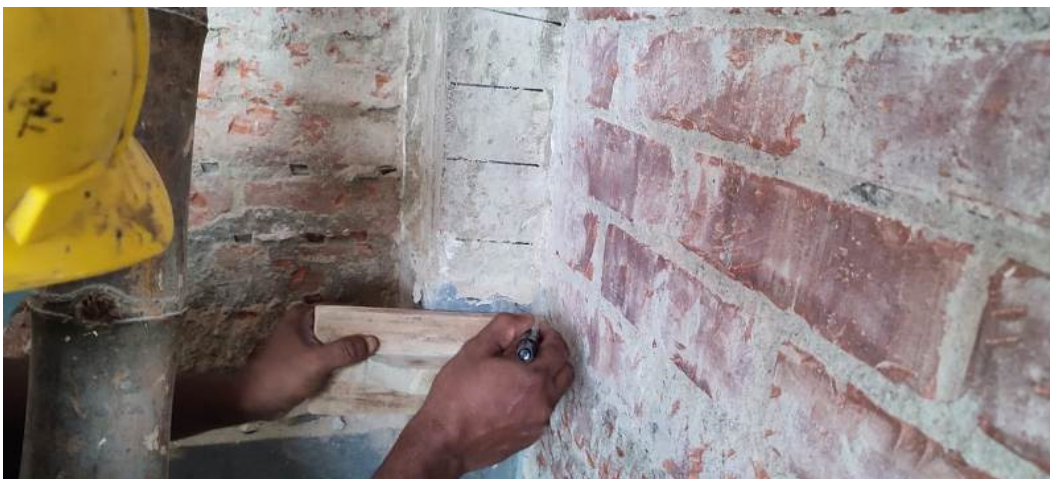
Figure A.2.8: Marking brick line to install nail
