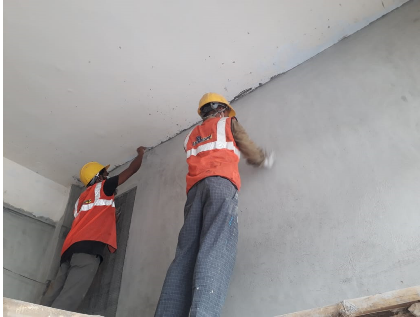
Figure A.2.67: First coat paint work for paint work
