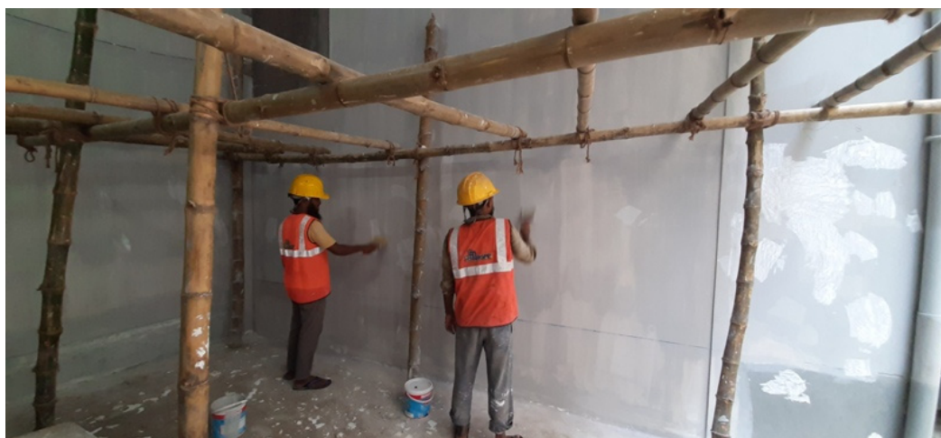
Figure A.2.69: Final coat paint work
