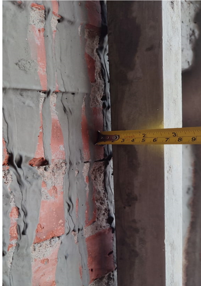
Figure A.2.42: Checking the thickness of mortar work
