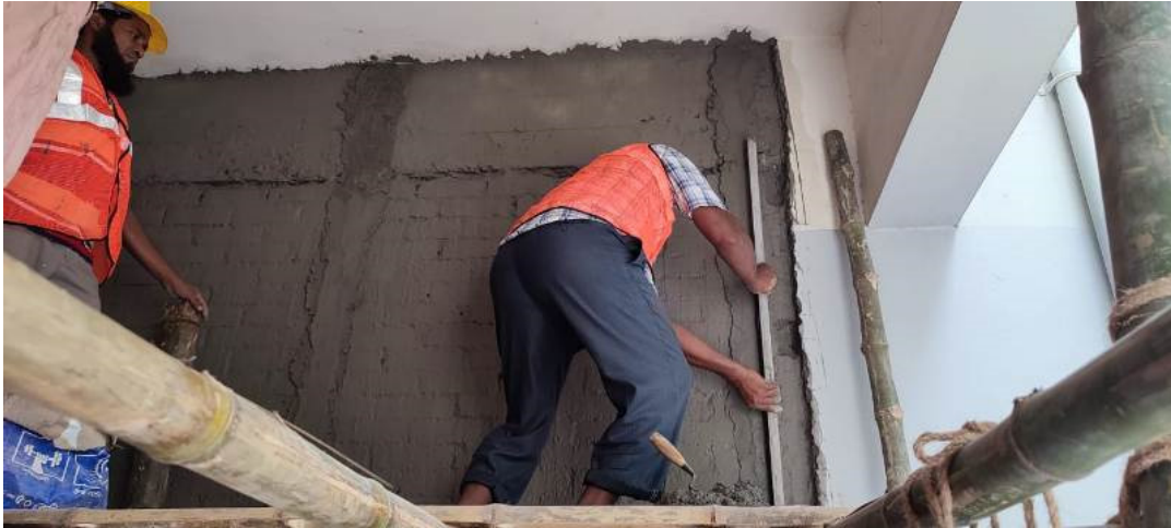
Figure A.2.40: 8 mm first layer mortar work (locally known as rough plaster)
