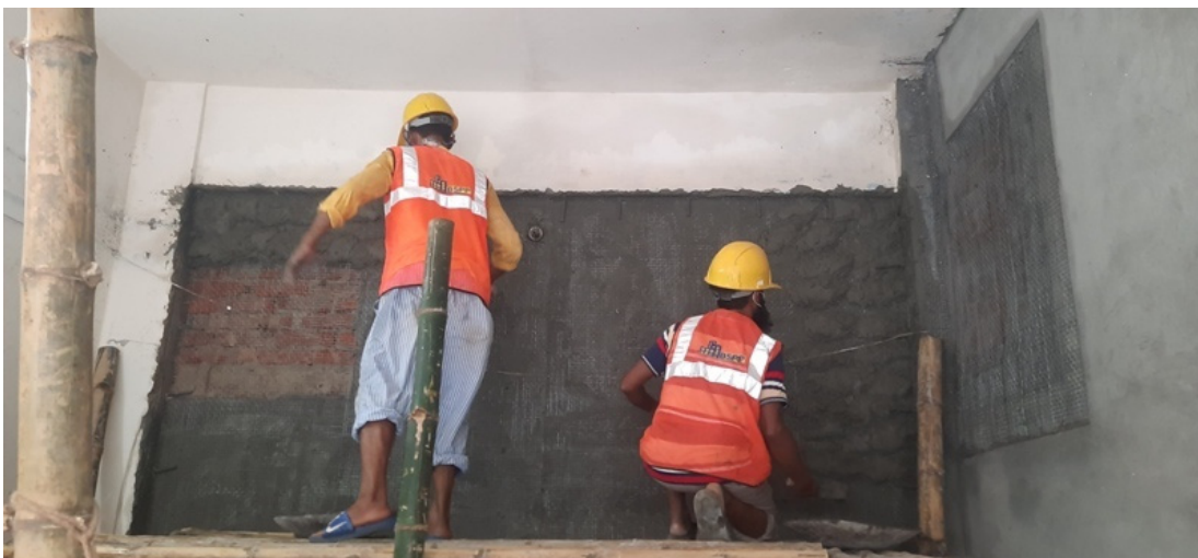
Figure A.2.26: 2 nd Phase mortar work with wire mesh (20 mm)
