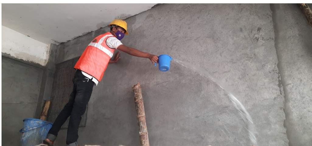
Figure A.2.65: Spreading water for curing work (7 days) to avoid crack
