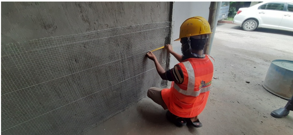
Figure A.2.43: First layer wire mesh installation (horizontal laying)
