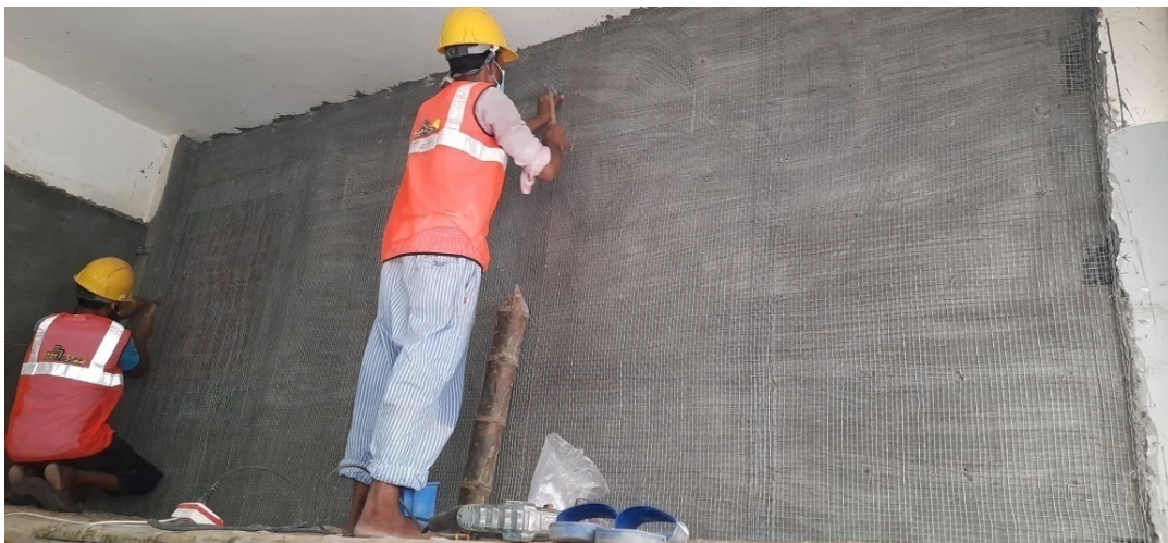
Figure A.2.51: Nail installation after wire mesh laying to avoid sag
