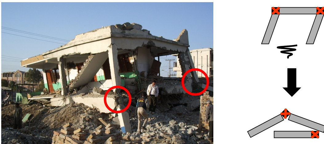
Figure C.1.4 Damage to beam-column joints, losing a building's integrity (2005 Kashmir earthquake)
