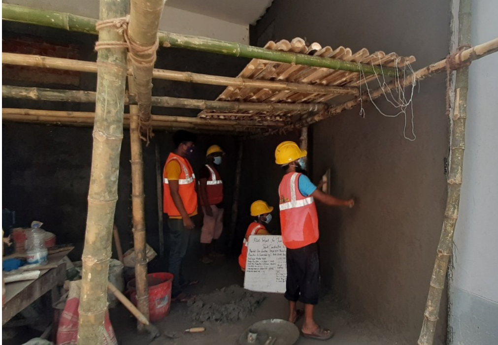
Figure A.2.47: 8 mm second layer mortar work with wire mesh
