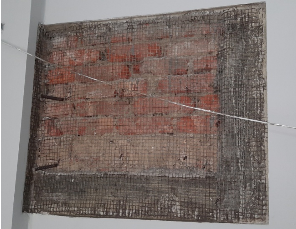
Figure A.2.33: Display of different layer of mortar work for SATREPS- TSUIB, Bangladesh portion, Wall-A
