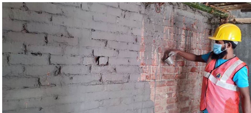
Figure A.2.9: Cement grouting work
