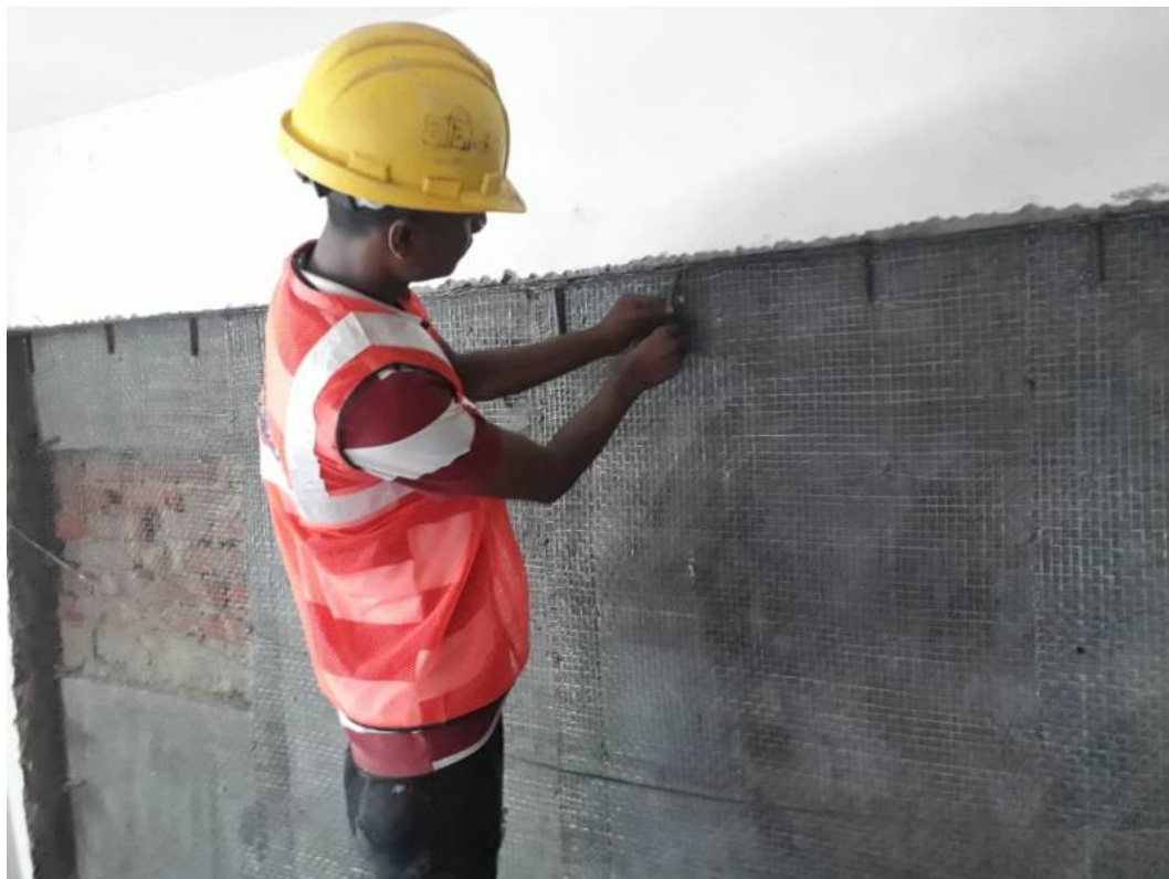
Figure A.2.23: Installation of dowel with epoxy resin/ Anchoring work
