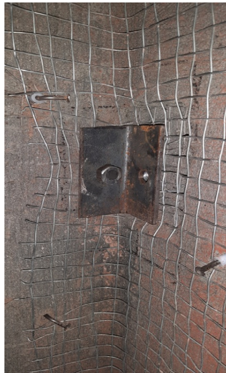
Figure A.2.58: Angle, rawl bolt and nut bolt installation to connect existing brick and column with wire mesh. Head of nut is removed after installation if required.
