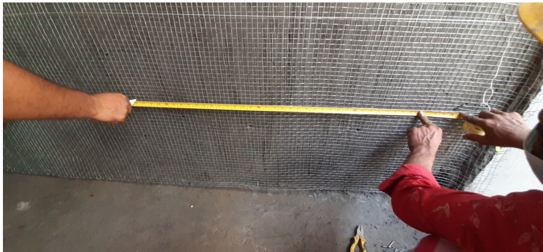
Figure A.2.45: Marking the point for installation of nail
