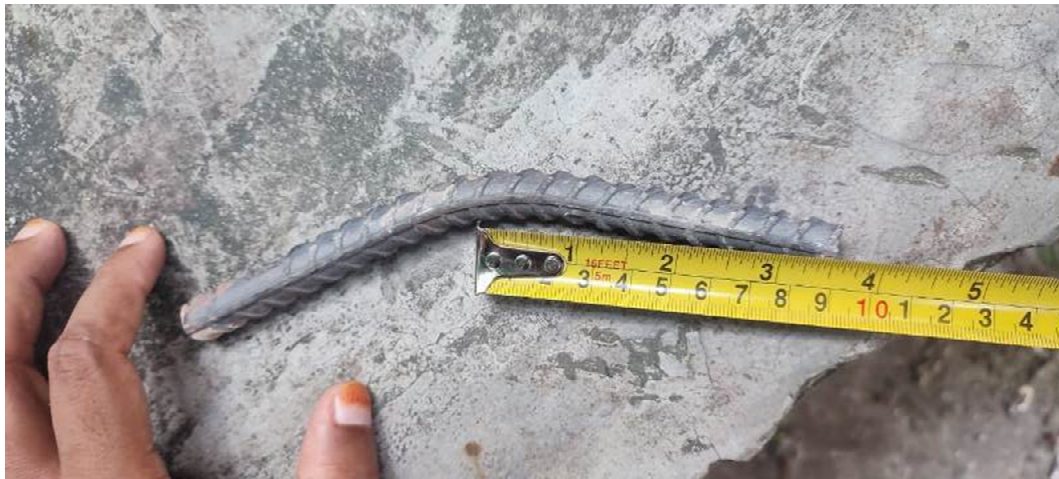
Figure A.2.22: Preparation of dowel before installation (bending as per design)
