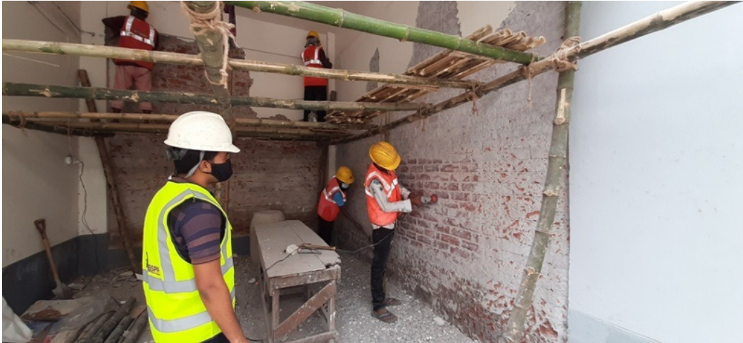
Figure A.2.37: Cleaning the brick surface
