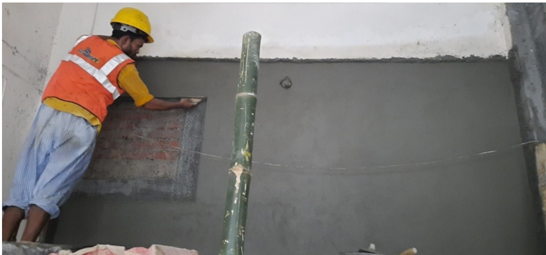
Figure A.2.28: Finishing the final phase mortar work
