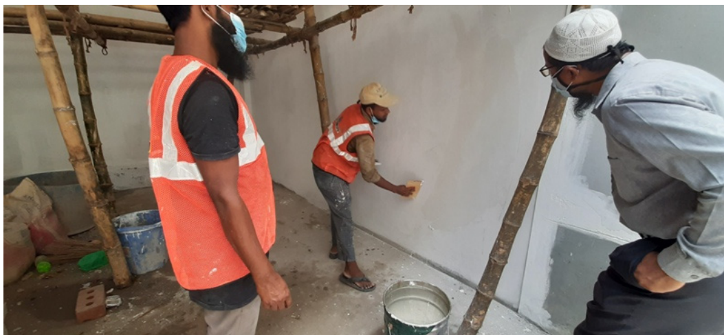
Figure A.2.68: Final coat paint work
