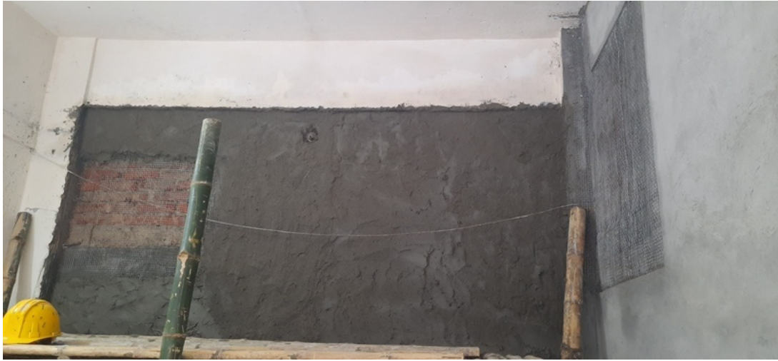
Figure A.2.27: 2 nd Phase mortar work with wire mesh (20 mm)
