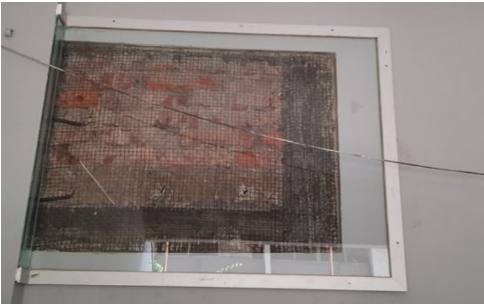
Figure A.2.34: Display of different layer of mortar work for SATREPS- TSUIB, Bangladesh portion, Wall-A
