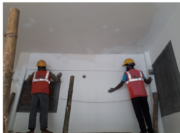
Figure A.2.32: Final coat paint work
