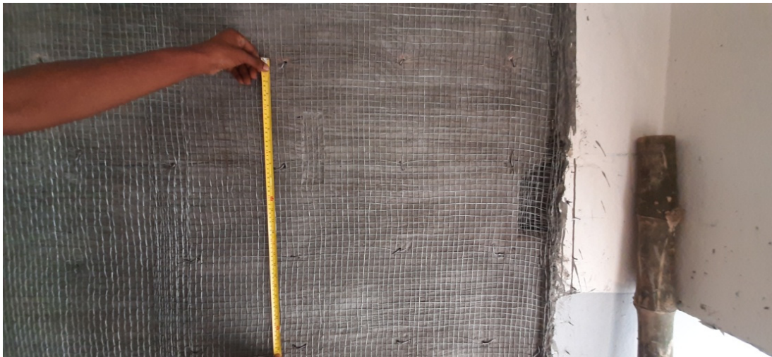
Figure A.2.53: Checking the distance of nail (vertical)
