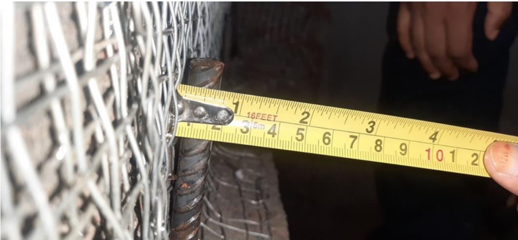
Figure A.2.25: Checking the minimum length required for final mortar work to cover dowel.
