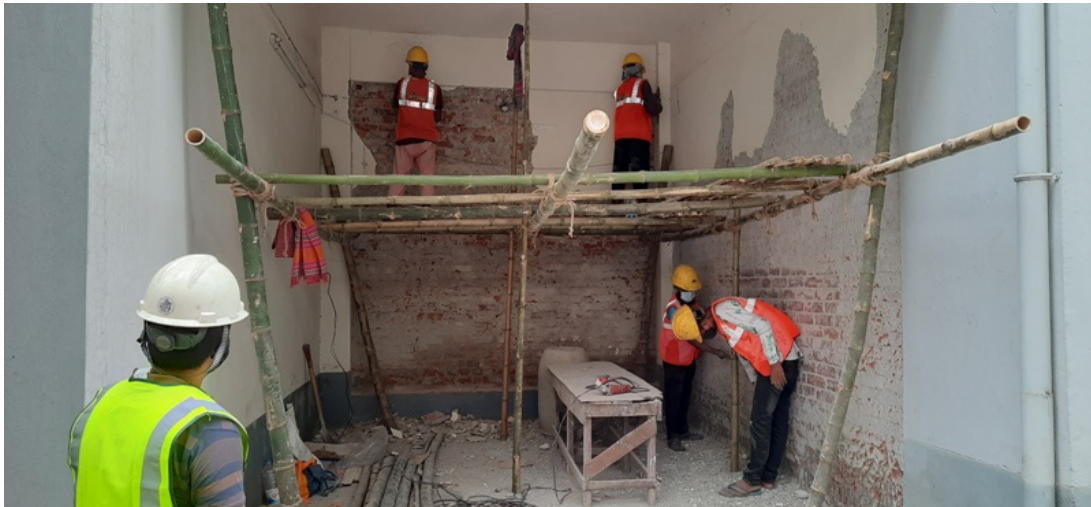
Figure A.2.4: Plaster removal for existing brick wall
