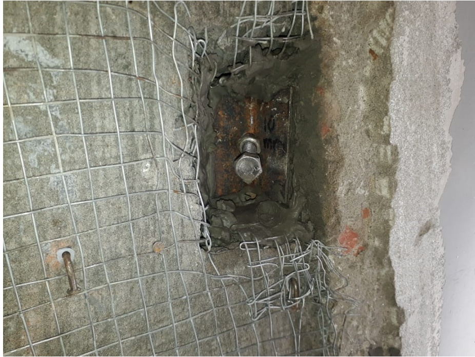
Figure A.2.59: Angle, rawl bolt and nut bolt installation to connect existing brick and column with wire mesh.
