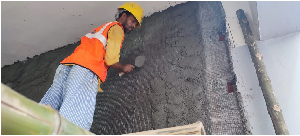
Figure A.2.62: Final (3 rd ) layer mortar work with second layer wire mesh
