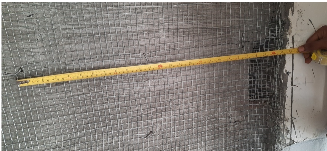
Figure A.2.54: Checking the distance of nail (horizontal)
