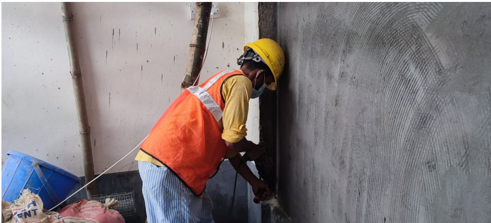
Figure A.2.14: Drilling work for dowel installation (downward)
