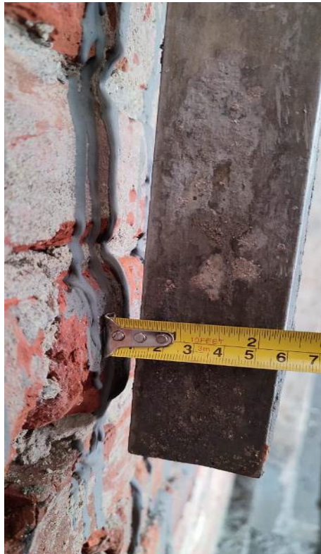
Figure A.2.11: Checking the thickness of rough plaster
