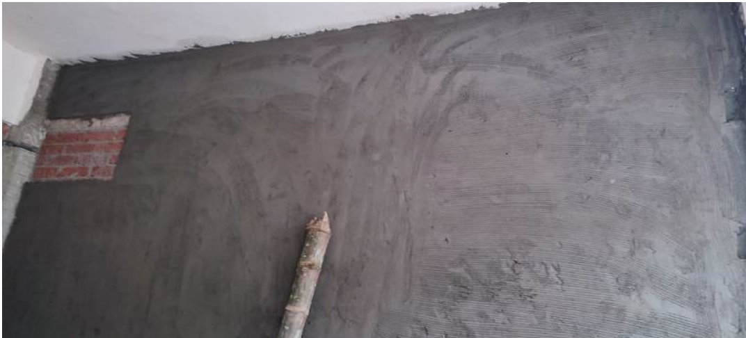
Figure A.2.41: 8 mm first layer mortar work (without wire mesh)
