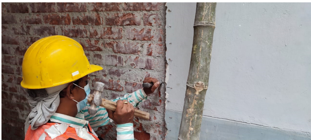
Figure A.2.39: Marking and cleaning the existing brick line
