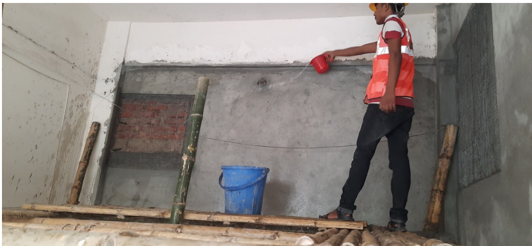
Figure A.2.30: minimum 7 days curing to avoid any form of crack
