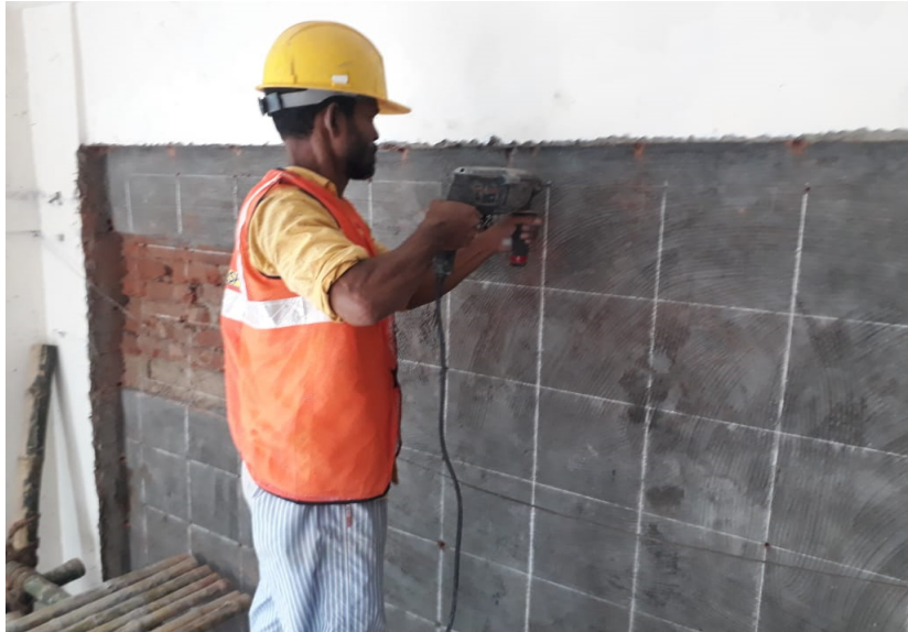
Figure A.2.13: Marking and drilling work for nailing
