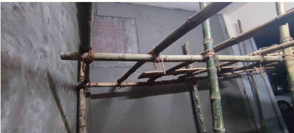
Figure A.2.63: Completion of 10 mm final layer mortar work
