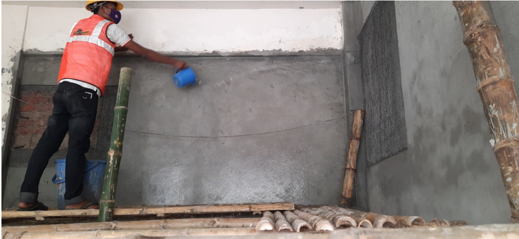
Figure A.2.29: Spreading the water for curing work
