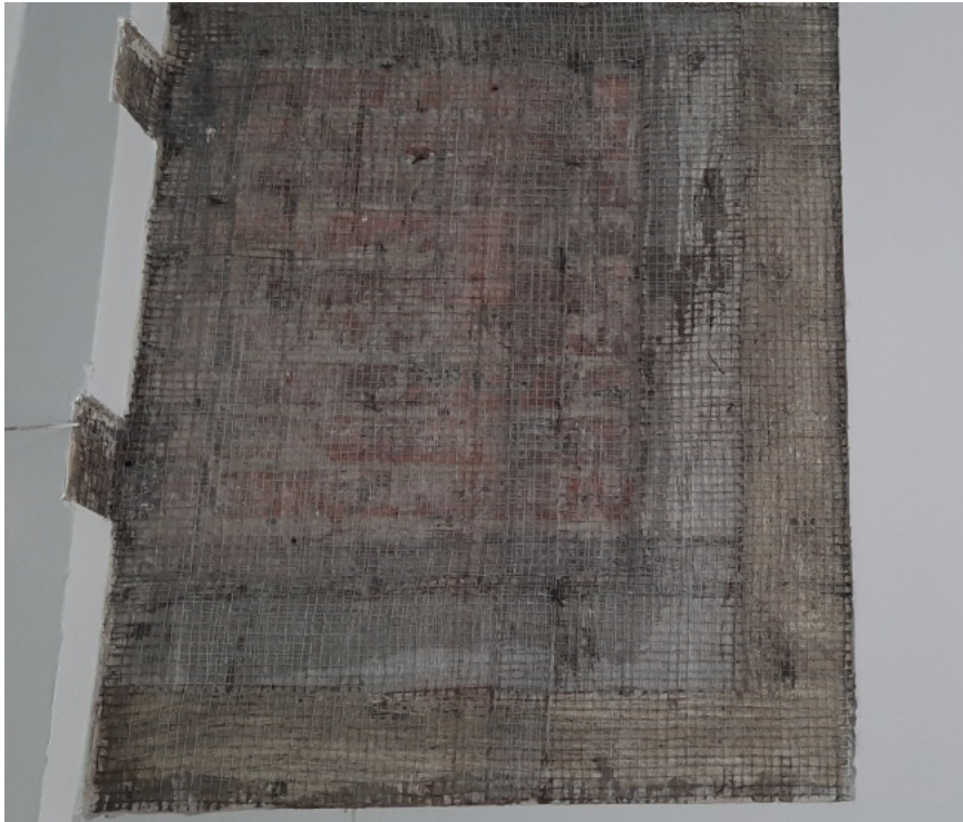
Figure A.2.70: Display of different layer of mortar work for SATREPS-TSUIB, Wall-A
