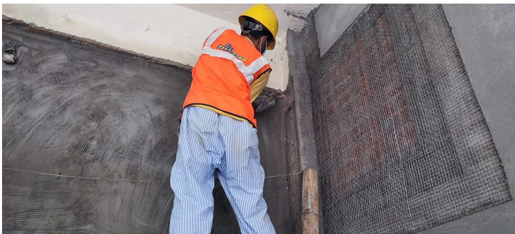
Figure A.2.15: Drilling work for dowel installation (upward)
