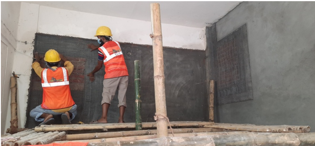
Figure A.2.17: Wire mesh installation
