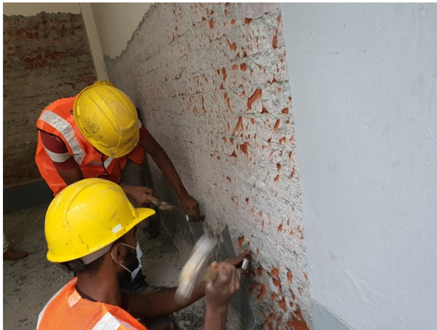
Figure A.2.36: Removing brick joint plaster
