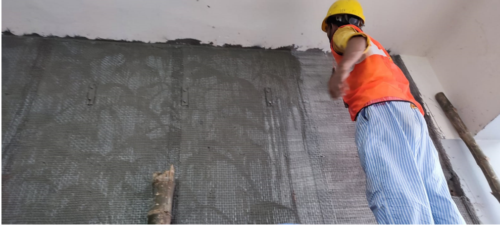
Figure A.2.61: Cement grouting spreading for final (3 rd ) layer mortar work
