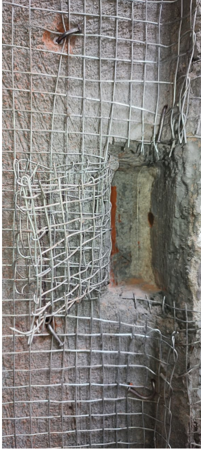
Figure A.2.49: Drill work to install angle, rawl plug and nut bolt if thickness of mortar work cannot cover the width of angle
