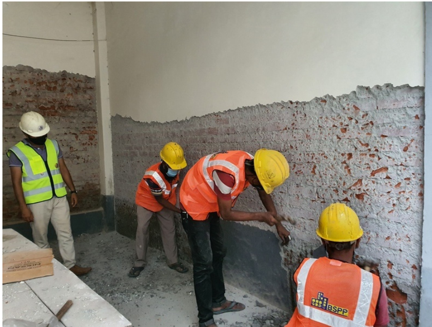
Figure A.2.35: Removing existing plaster work of brick wall
