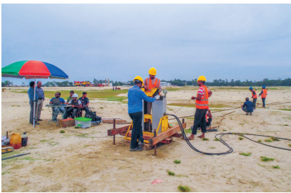
Cone Penetration Test
