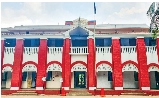
Dr. M. A. Rashid Administrative Building
