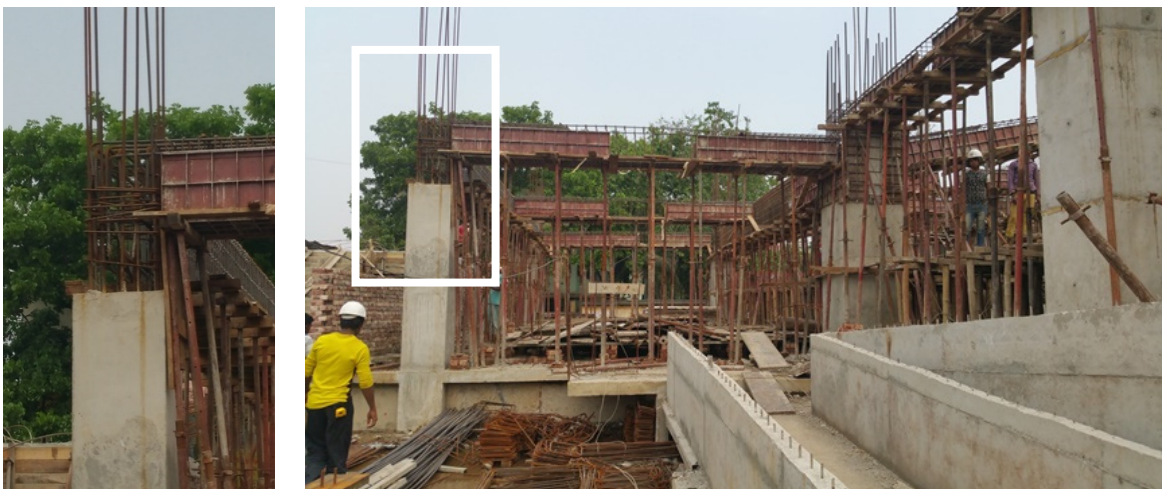
Figure C.5.1 Typical exterior beam-column joint under construction in 2017.
