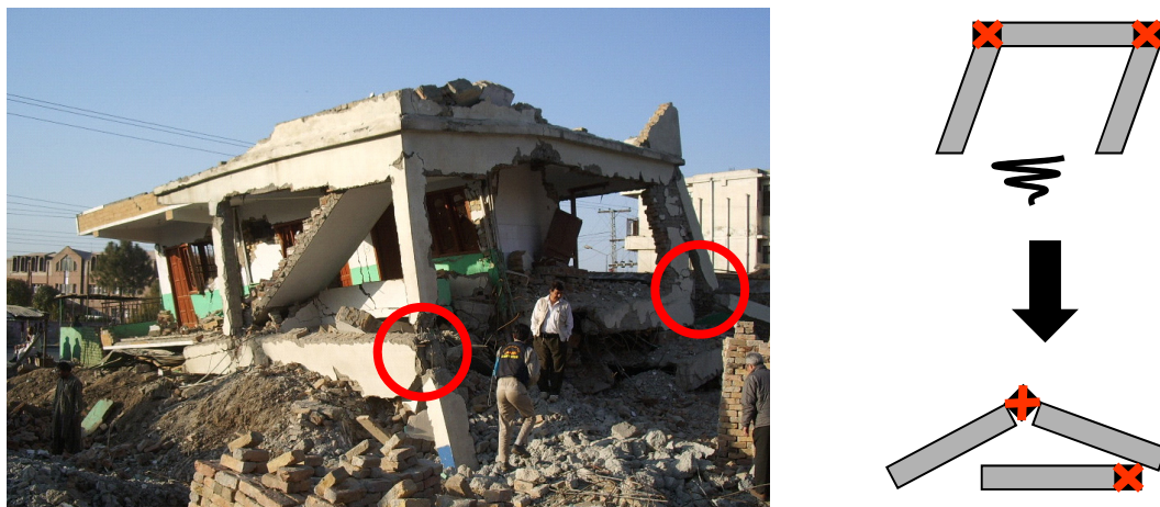
Figure C.1.4 Damage to beam-column joints, losing a building's integrity (2005 Kashmir earthquake)
