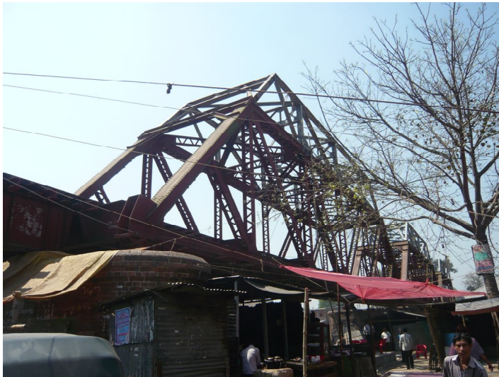
Figure 7. Boral bridge after installation of new top chord bracing system.
