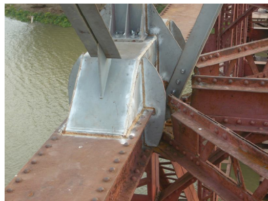
Figure 9. A view of the new top chord bracing system after installation above the old bracing system.
