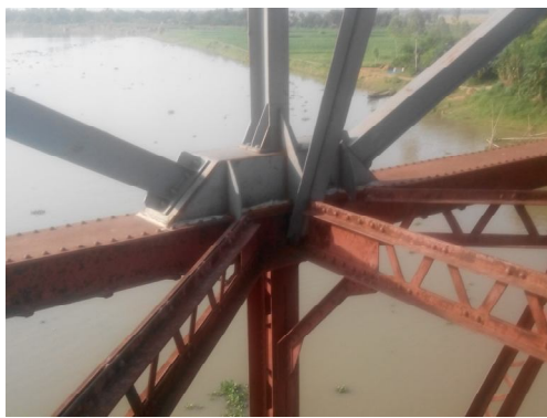
Figure 9. A view of the new top chord bracing system after installation above the old bracing system.
