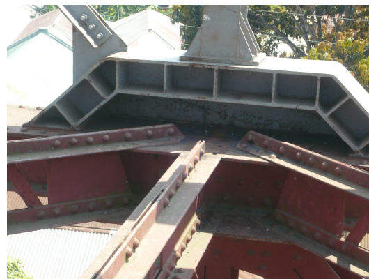
Figure 10. Details of under-construction connection between the existing top chord and the new member
