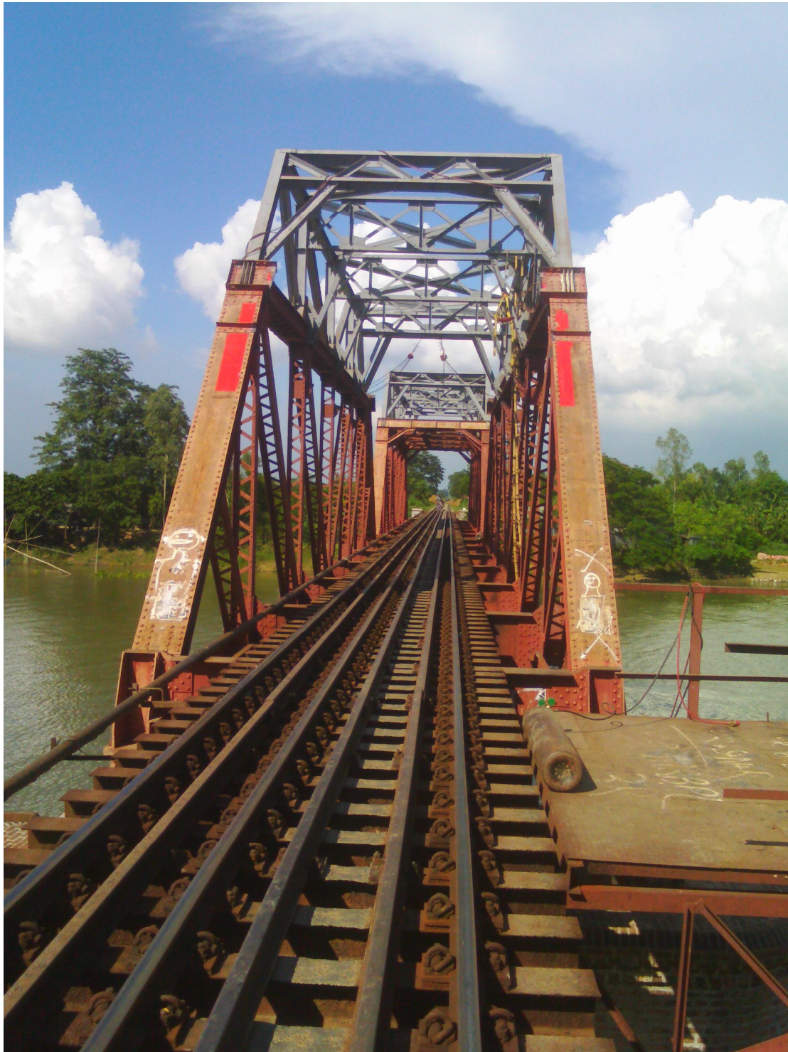
Figure 8. Koidanga Bridge after instillation of the new top chord bracing system.
