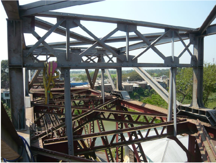
Figure 9. A view of the new top chord bracing system after installation above the old bracing system.
