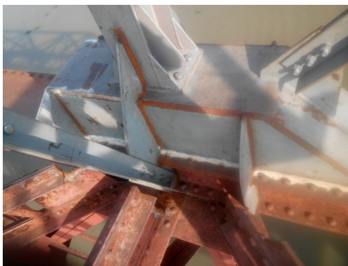
Figure 10. Details of under-construction connection between the existing top chord and the new member
