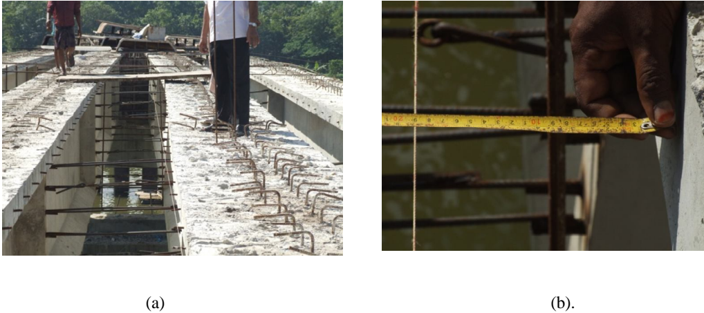
Figure 1. Girders seen from the top. (Left to Right: 2A, 2B, 2C, 2D. (a) The lateral deflection of the girder 2C is visible. (b) Lateral deflection of the Girder 2C seen at the top near the mid span
