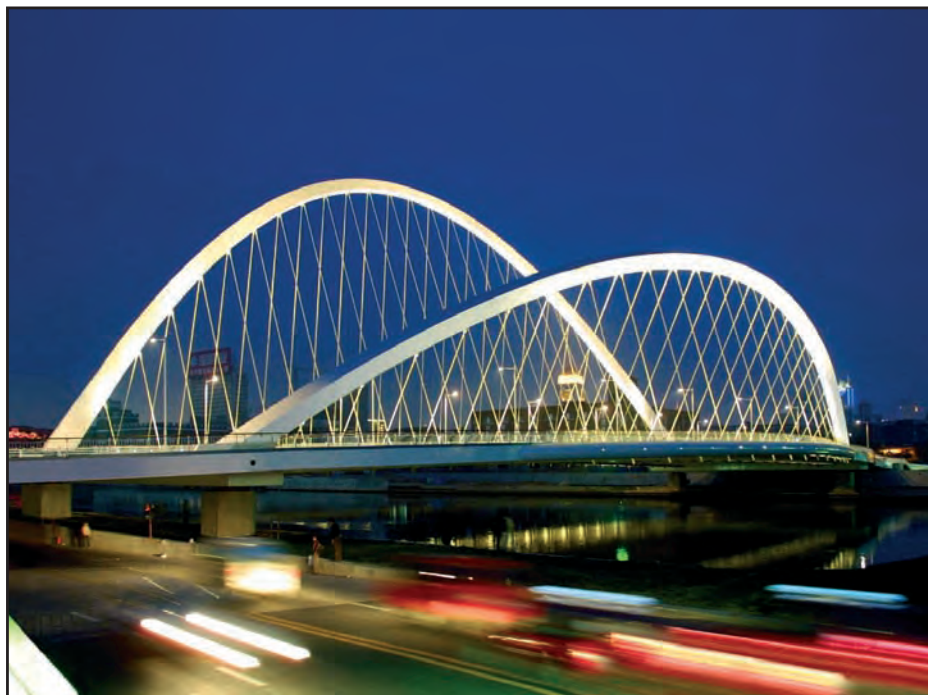
Dagu Bridge, Tianjin, China
